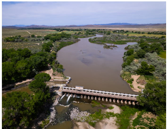
Aerial view of Carson River Diversion Dam.
